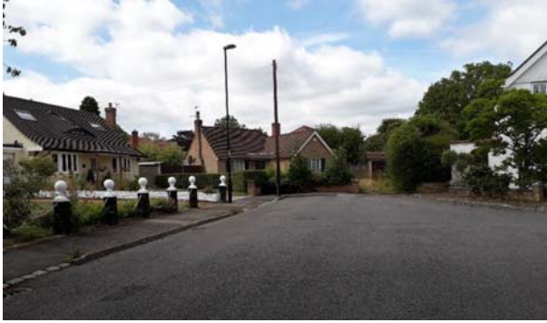
From Kearton Close (facing the site)
